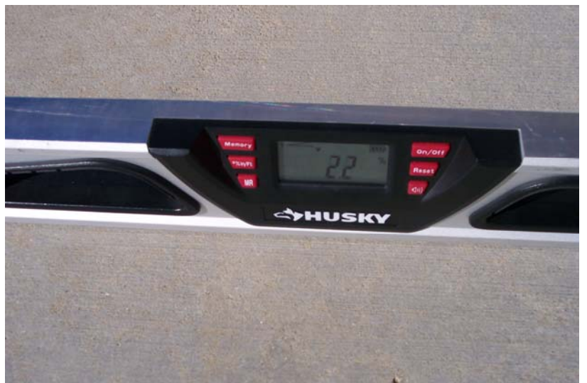
C2. POT from South Accessible Parking Sidewalk Slope to Front Door
