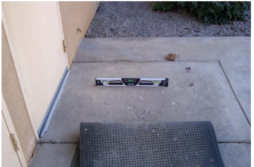
K3. Rear Exit to North Parking Trash Enclosure
