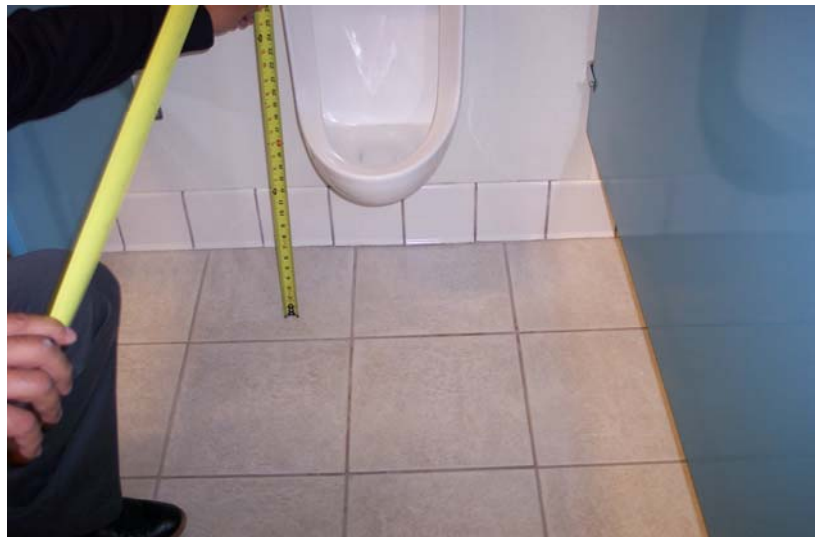
B1. Men's Restroom Urinal
