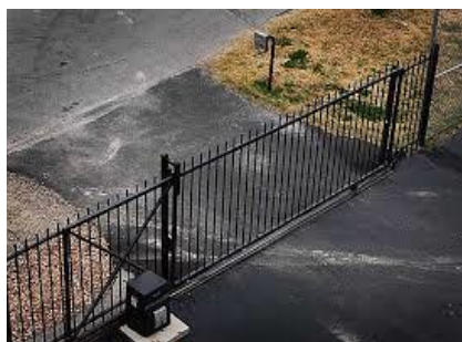
Controlled Access w/perimeter fence
