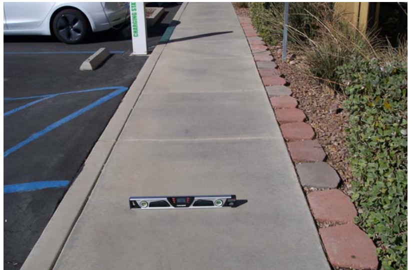
C1. POT from South Accessible Parking Sidewalk to Front Door
