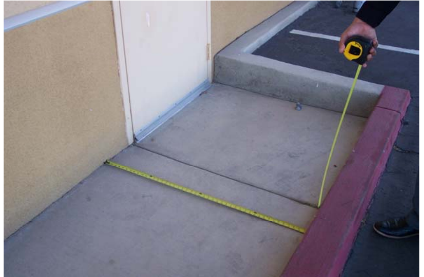
L2. West Exit Door Landing
